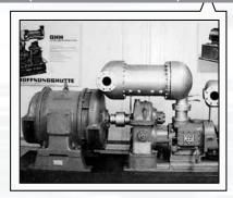
1952 The world's first oil-free rotary compressor is introduced
