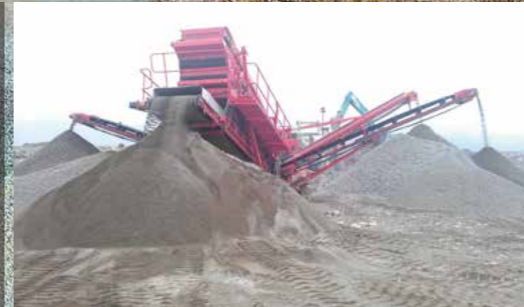
NFS350's application of the pebble and rover sand screening of riverway in Gansu Province
